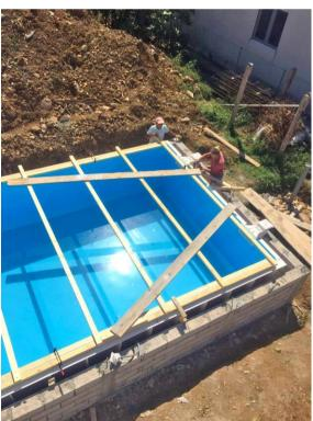
When is properly fixated (which can be inspected by visual check) the swimming pool can be filled with water. When pool is filled with 30-40cm of water, then concreting of the space between walls of the construction hole and walls of the swimming pool with dry concrete can start.
